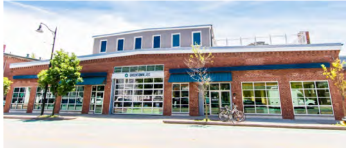
Photo : Greentown Labs
